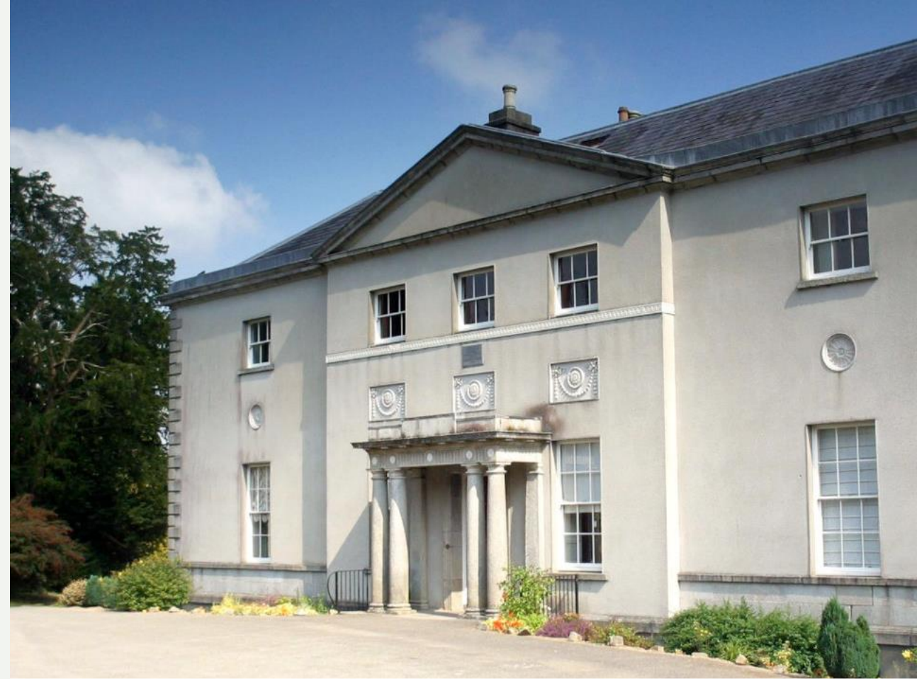
Fig. Avondale House, Co Wicklow
